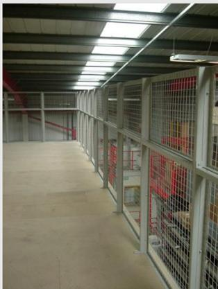
A mesh wall system designed to protect personnel while in hazardous areas. This product can work in combination with the solid partitioning and our pedestrian safety barrier system, demonstrating the versatility of both systems.
