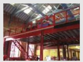
A Barrier System designed to create safe pedestrian areas both on ground and on mezzanine floors.
